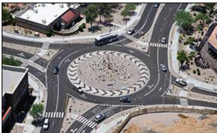
Road merging into a roundabout (circular road)
